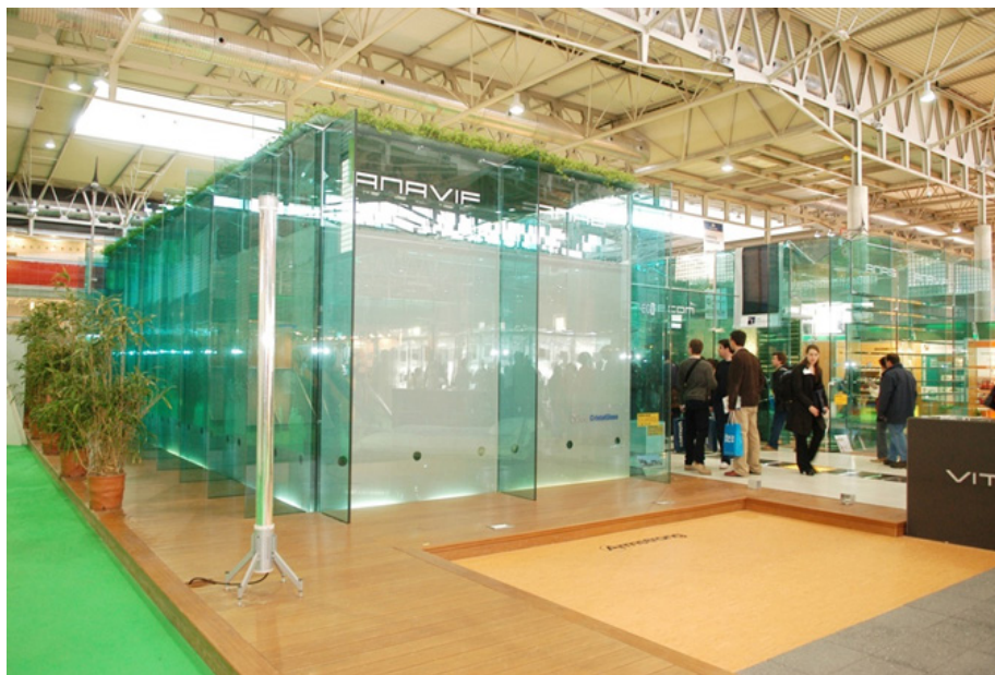
Figure 7: Vitrohouse's architectural envelopes are highly varied and include a triple glass skin with two air chambers: a sealed inner chamber and a ventilated outer chamber. The outer chamber includes blinds that regulate sunlight from zero to 100%
