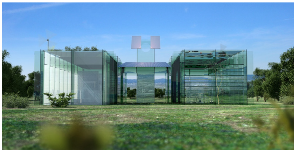
Figure 4: The Central Roof of Vitrohouse Is Composed of Two Layers of Flat Glass and Integrates Solar Panels on Its Exterior, Which in Turn Provide Thermal Insulation and Solar Protection to The Interior
