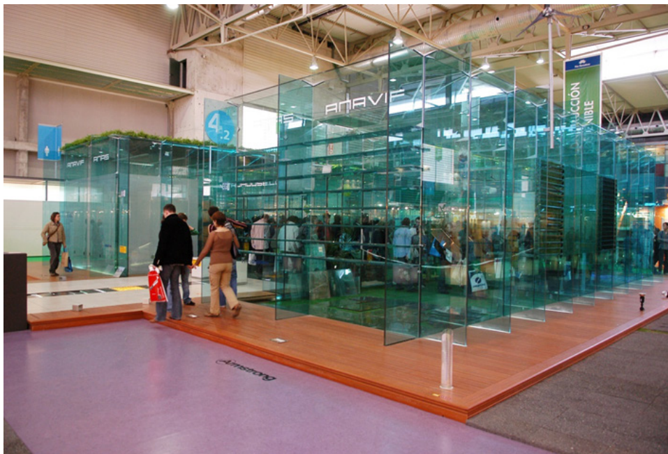
Figure 9: The Right side of Vitrohouse is Completely Transparent, and Thermal Insulation is Achieved by Injecting Hot or Cold air into the Triple Skin of the Architectural Envelope. The air is Drawn in from Inside the House as it is Renovated
