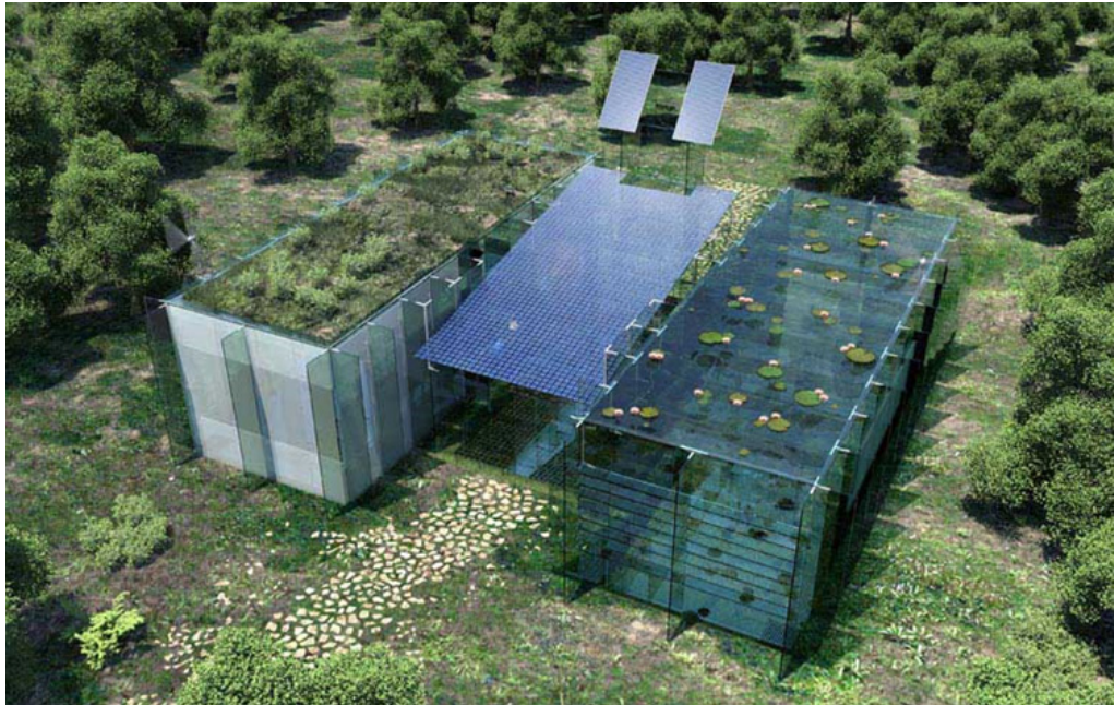
Figure 1: Vitrohouse Was Built Using Only Removable Components Made of Flat Glass (Project by Luis De Garrido)
