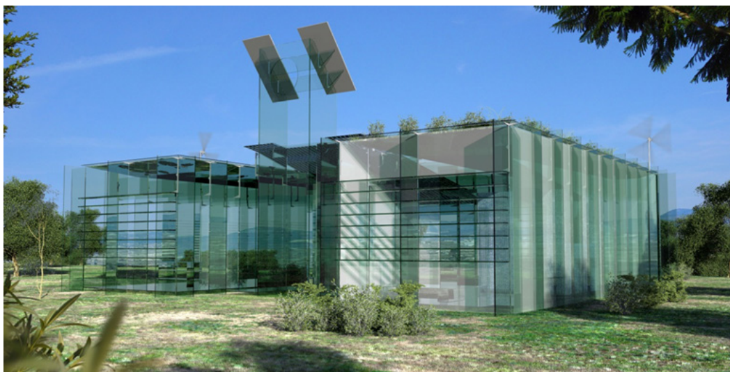
Figure 2: Vitrohouse is an Energy-Self-Sufficient Home that Integrates Fresh Air-Capturing Chimneys, Solar Thermal Collectors, and Photovoltaic Solar Collectors (Project by Luis De Garrido)
