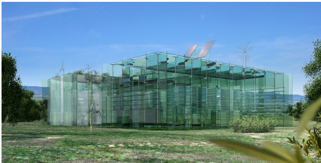
Figure 3: Vitrohouse Integrates Green Roofs, Water Roofs, and Vertical Gardens Despite Being Built with Glass
