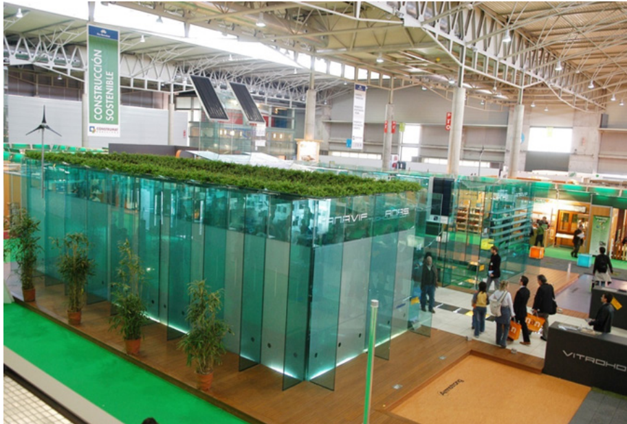
Figure 8: The Left Side of Vitrohouse Incorporates Glass whose Opacity Changes Through Small Electric Currents, Regulating Privacy and Solar Protection
